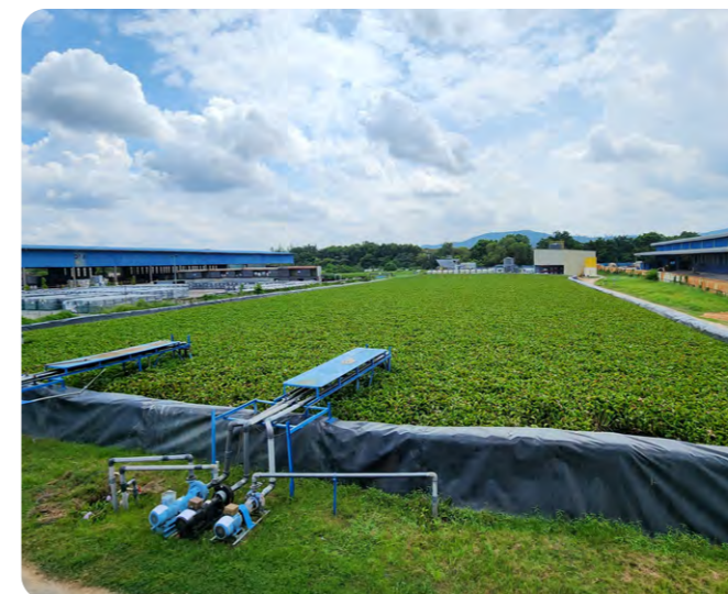
Water hyacinth is planted as a phytoremediation plant to reduce iron concentration in the water
